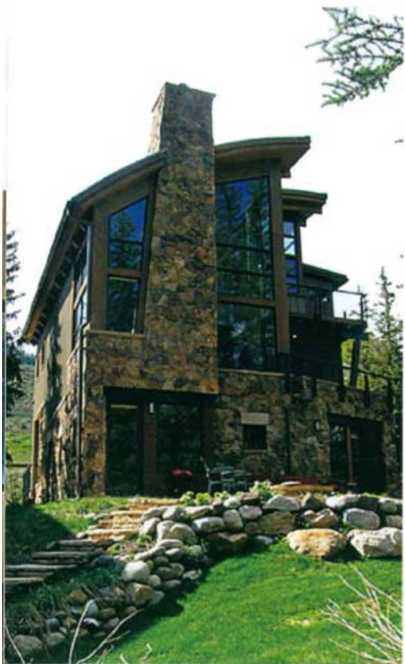
A one-piece, curved metal roof is just one of the many distinctly modern, high-tech features of the Kalstrom residence in West Vail.
